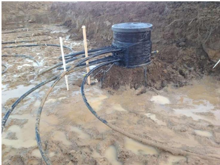
*Manifold chamber with lid prior to back-filling*
