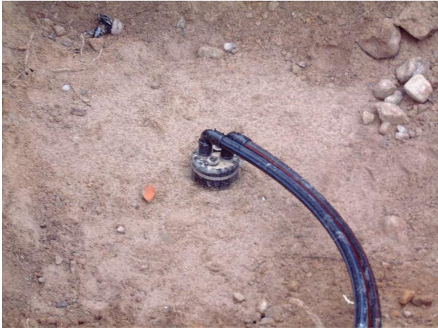
*Neoprene borehole sealing cap*
