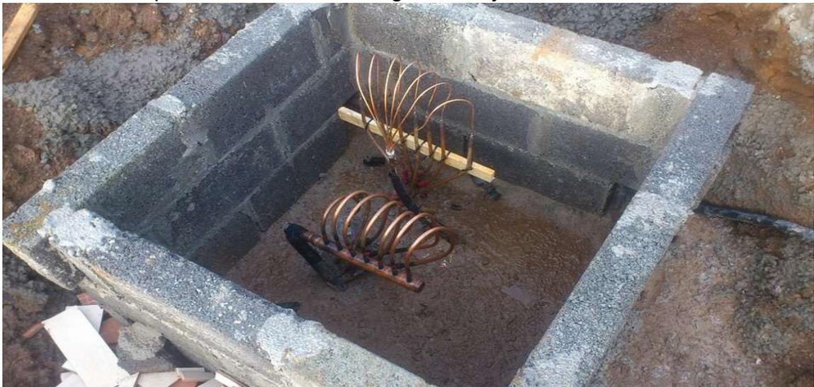
8. The pipe to the distributor should rise vertically with at least 200mm of straight pipe before entering the distributor to allow even distribution of the refrigerant through all collector pipes. It is also desirable that each distributor tail be at least 500mm long for the same reason.
