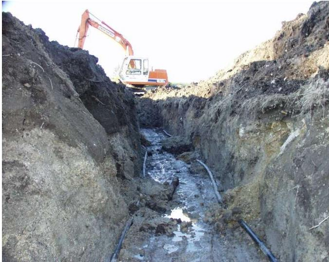
Care must be taken that the collector piping is laid joint free in continuous rolls and obviously free from contact with sharp rocks or stones before back-filling.
